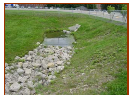
Picture showing forebay
