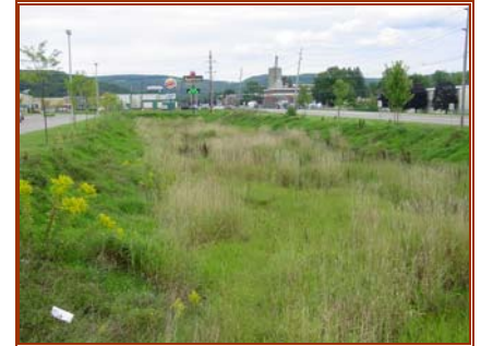
Picture showing infiltration basin
