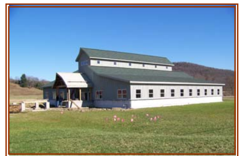
Education Center/Office Complex under construction
