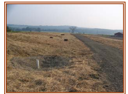
Stabilized laneway, basins, and waterway just after construction.
