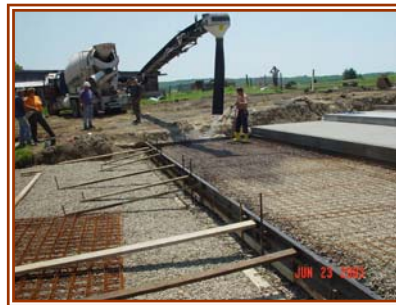
Concrete stairs during construction.
